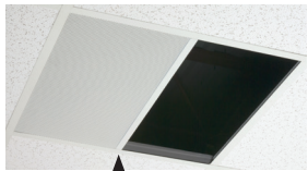
Integral T-bar supports neighboring non-regular tile.
