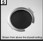
Use a saw to cut the hole. For a drywall ceiling, the support rails provided need not be used, but it is recommended that the "C ring" be used to support the cut-out edge of the drywall. The gap in the C-ring allows the ring to be maneuvered into position as shown. Install so the dog ears rest on the ring.
