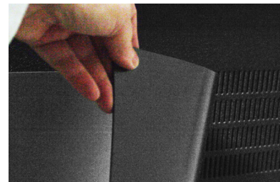
Magnetic vent blockers are typically installed inside the rack to cover vents near the top of the rack. When a fan panel is installed in the rack top, air can be drawn through (open) vents at the bottom, past the covered vents and exhaust through the fan panel.
